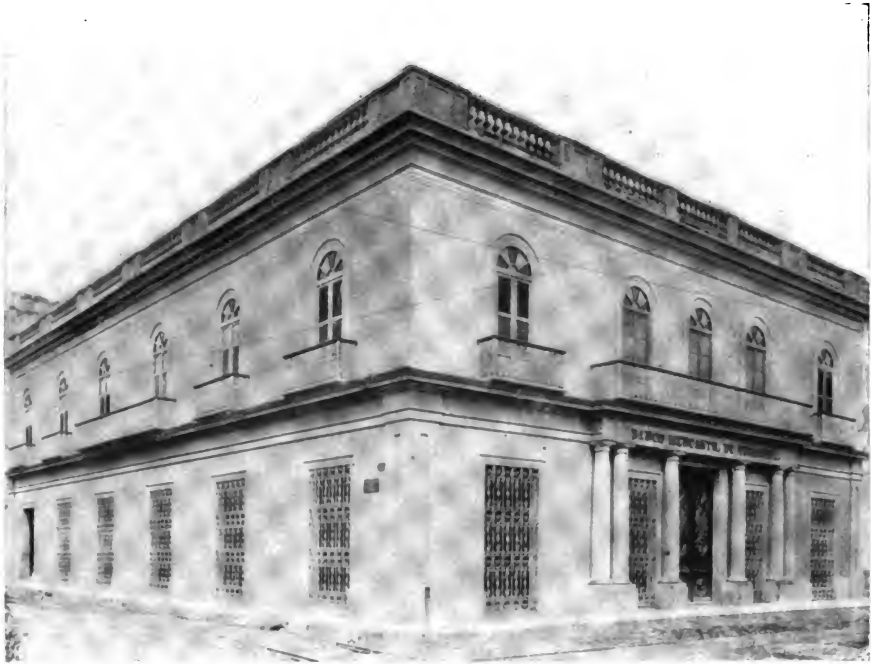
Exterior of Bank Building.
